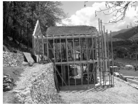
Fig. 17. Building in process
