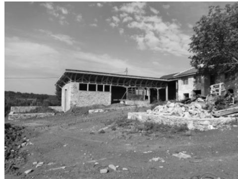
Fig. 22. The renovated barns and farms
