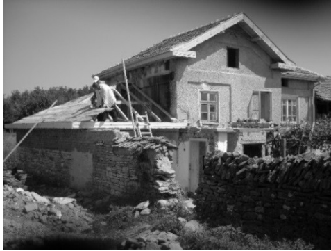
Fig. 10. Village of Karpachevo, Lovech District – renovation of country house in process
