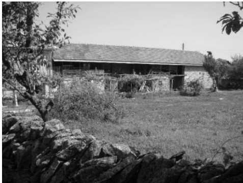
Fig. 12. In most cases repairs start with the roof
