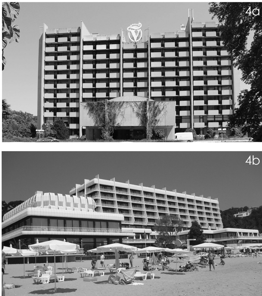
Fig. 4. Druzhba Resort Complex: (a) Grand Hotel Varna, arch. Georgi Ganev; (b) House 6 of complex of the Central Committee of the Bulgarian Communist Party, nowadays Hotel Palas, arch. Milena Jordanova
