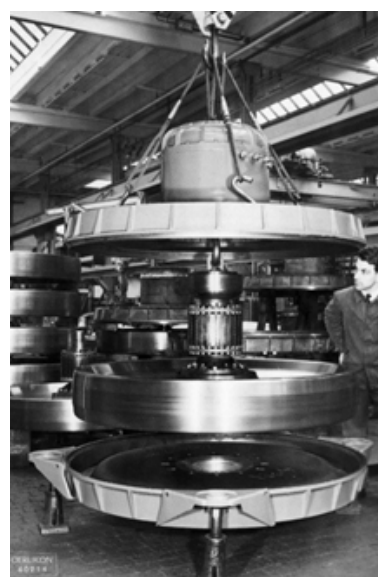
Fig. 4. Flywheel of the “Jyrobuss”
