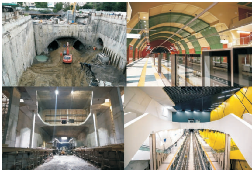
Fig. 14. Construction of MS Orlov Most under the modified NATM and view of the completed station. Construction of MS NDK 2 under the Top-down method and view of the station
