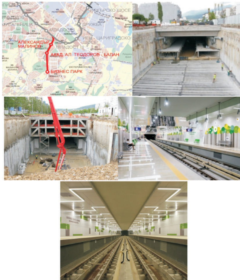
Fig. 7. Construction and view of MS Al. Malinov and MS Business park
