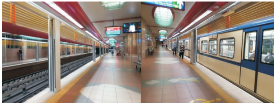
Fig. 12. Protective vertically opening screen doors between the platforms and the tracks (trains). These are installed at 12 of the busiest stations on Line 1
