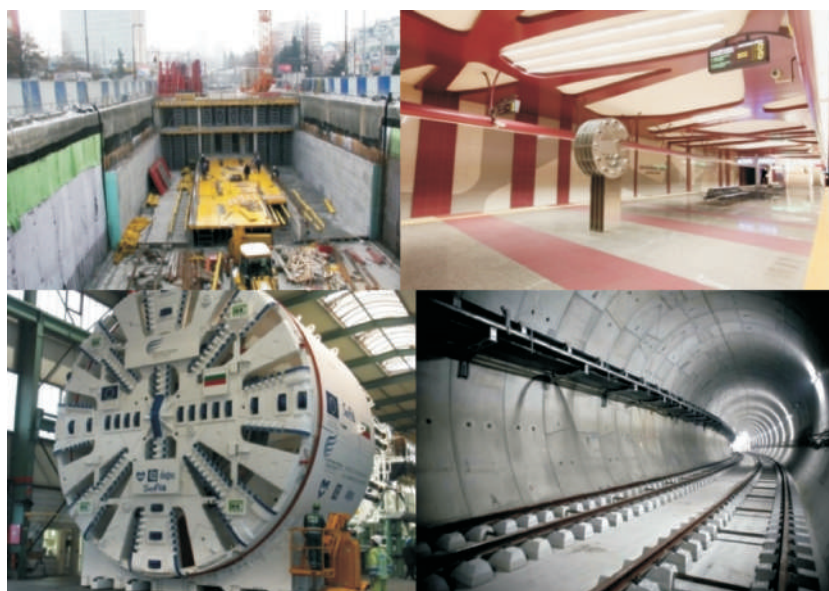
Fig. 10. Construction and view of MS European Union. Tunnel Boring Machine for the construction of the double-road tunnel and a view of the finished tunnel in the central section of Line 2
