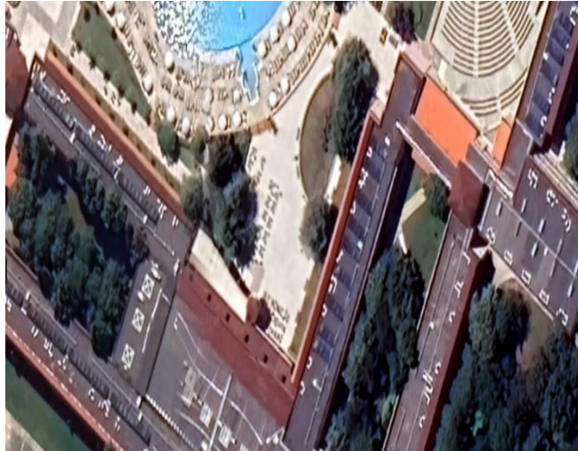
Fig. 1. Solar Collection System.
